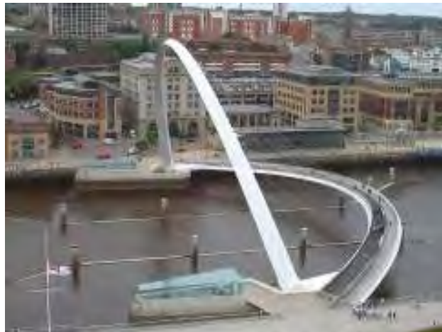
Examples of operable crossings
