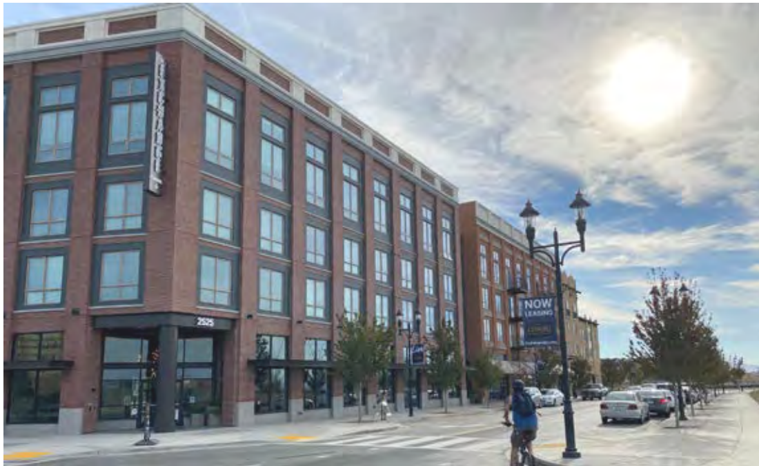
The top of the building is articulated with an entablature and parapet wall, Image source: www.719larkin.com
