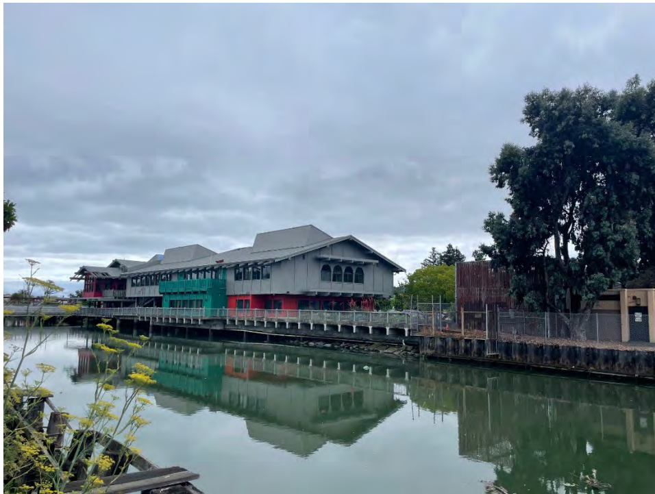
Canal Alliance Building (South Side of Channel)
