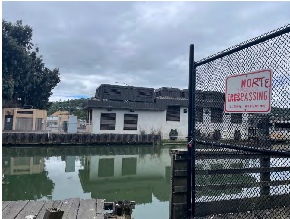
Municipal Building (Across Project Site, South Side of Channel)
